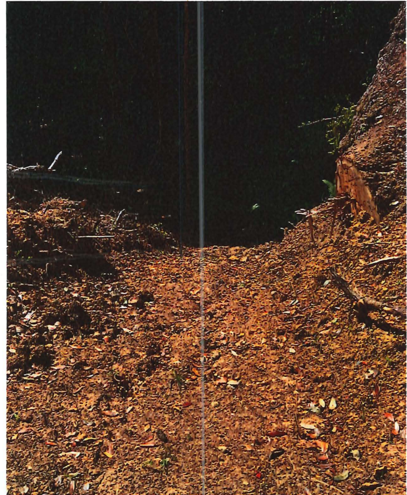
A severely eroded driveway on private land on the Hubbard Creek Watershed.
